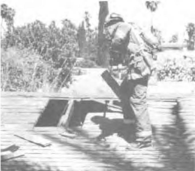
Fig. 29. Remove roof materials for the pullback
