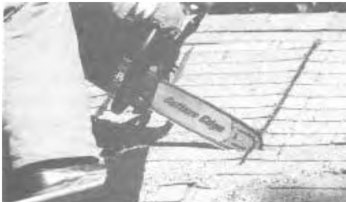
Fig. 26. Criss-cross, or overlap, your cuts.
