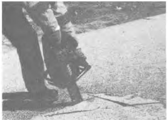
Fig. 27A. Inspection Cut.
