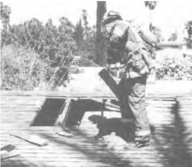
Fig. 24. Remove roof materials for the pullback.
